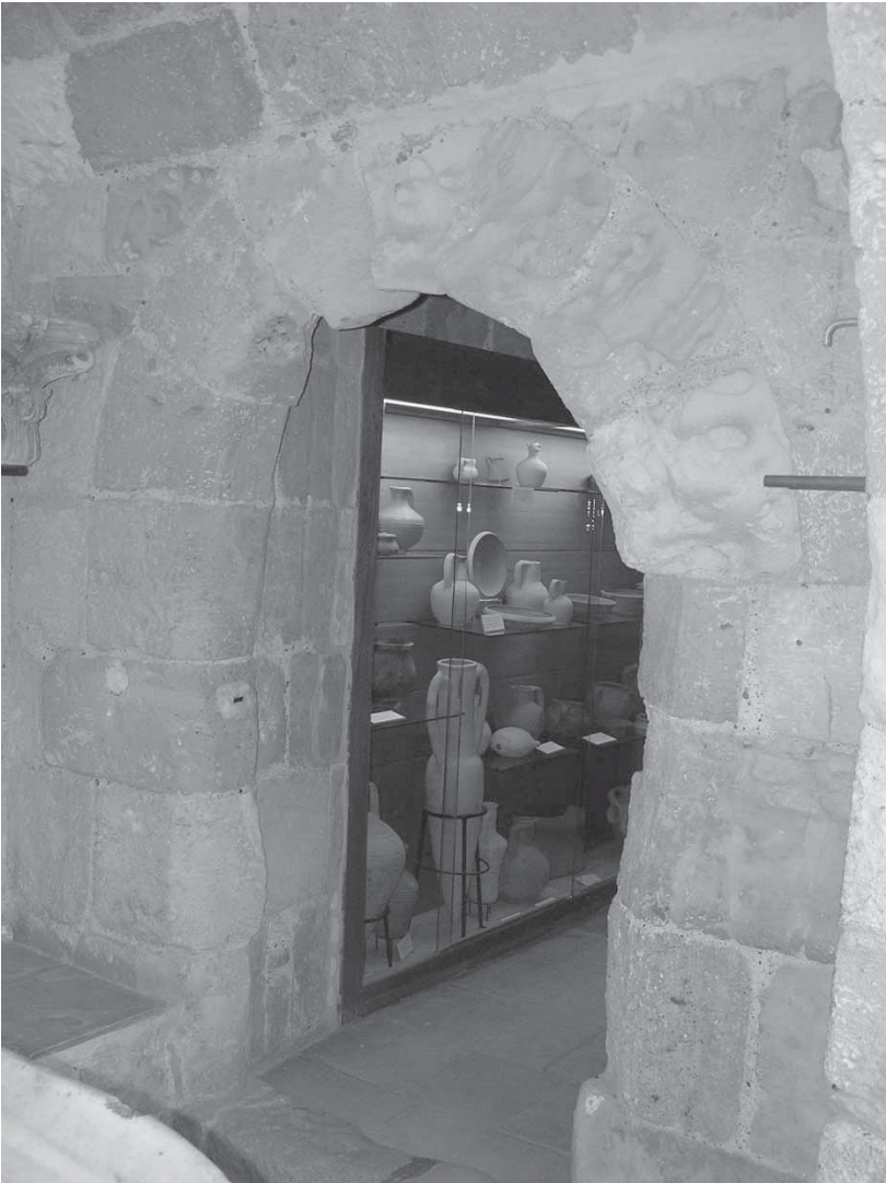
Fig. 33: Limassol Castle, upper level of cells, easternmost cell on south side, doorway showing signs of fire damage [M. Olympios].
